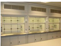
Re-circulation fume cupboard
