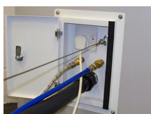
Mobile fume cupboard docking station
